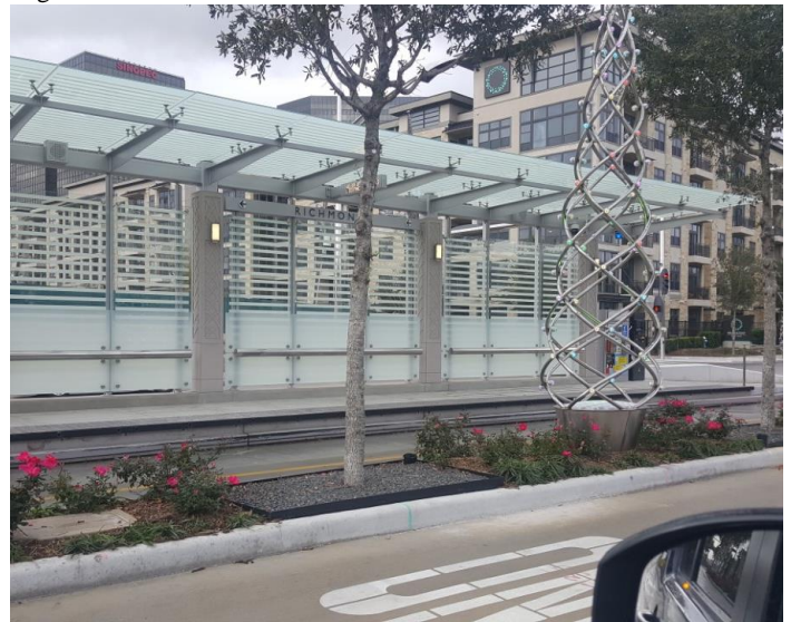
Richmond Ave stop on Post Oak's Silver Line, with curbs, covered shelter, landscaping, and lighting. A highly visible crosswalk with traffic lights is just out of view of this image, to the right of the shelter.
